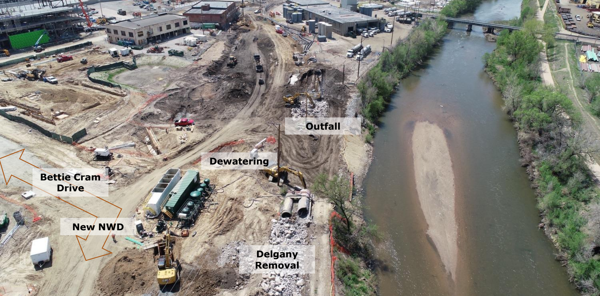
The intersection of Bettie Cram Drive and National Western Drive is taking shape as the Delgany Wastewater pipes are removed.
